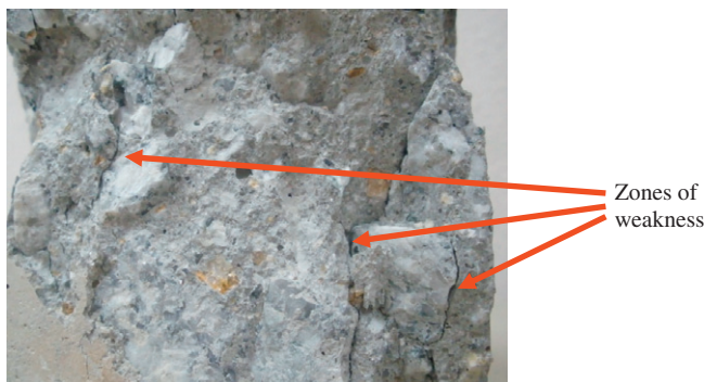
Fig. 5. Crack patterns of specimens.
