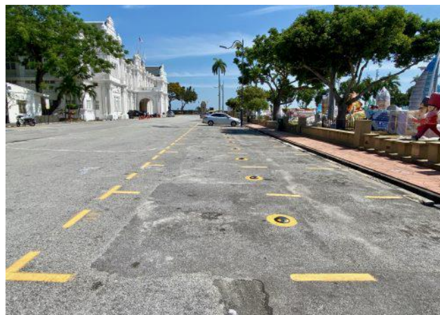
Figure 3. Location of magnetic sensors for the Penang smart parking system [6]
